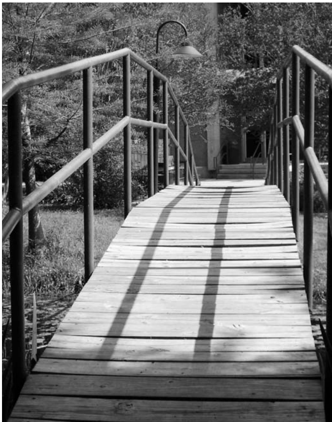
The bridge located behind the Science Building
